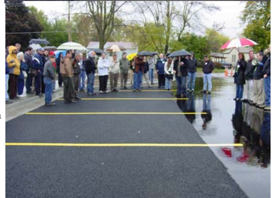
Above: Pervious Asphalt
